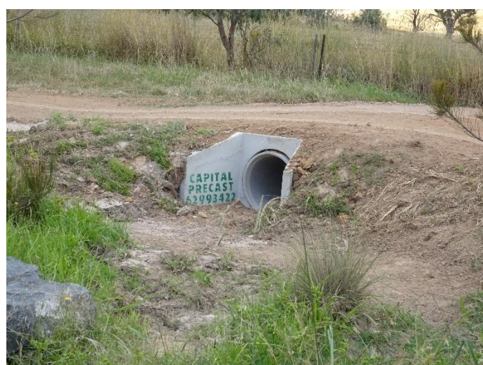
fitted culvert pipe photo Andy Russell
