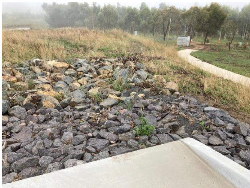
Drain which overflowed down into Forest 20 causing much damage.
