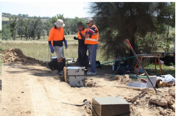
Foundations for the roof extension supports
